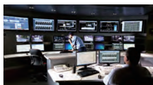
Command and control center
